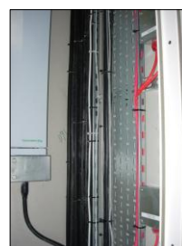
PHOTOGRAPH 11 TYPICAL RISER CONTAINMENT
