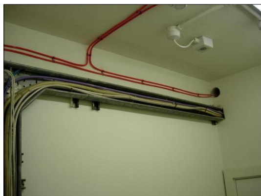
PHOTOGRAPH 7 HIGH LEVEL CONTAINMENT AND CABLE RUN ON LOWER GROUND FLOOR
