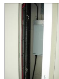
PHOTOGRAPH 12 TYPICAL RISER CONTAINMENT
