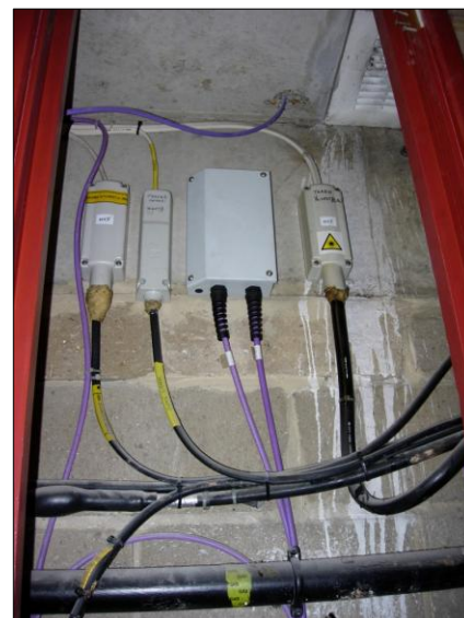
PHOTOGRAPH 6 EXISTING BT AND VODAFONE FIBRE SERVICES ADJACENT TO DUCT ENTRIES
