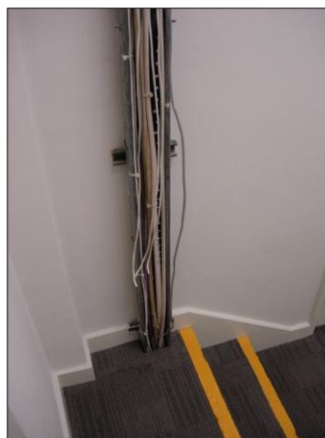
PHOTOGRAPH 8 CABLE ROUTE FROM HIGH LEVEL TO BELOW GROUND VOID ON LOWER GROUND FLOOR
