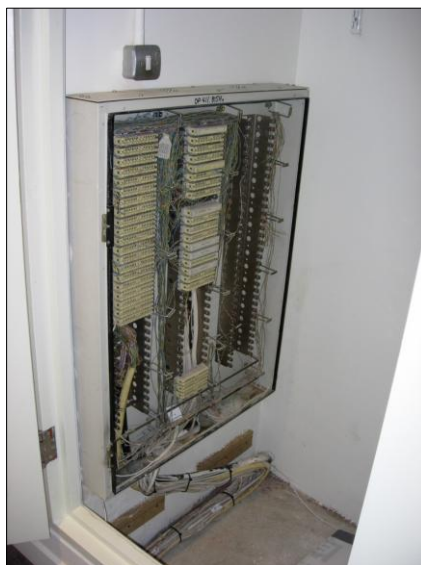
PHOTOGRAPH 5 EXISTING BT COPPER DISTRIBUTION POINT ON LOWER GROUND FLOOR
