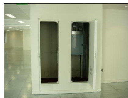
PHOTOGRAPH 10 TYPICAL MAIN RISER ON FLOORS
